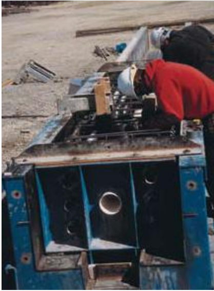
A moment-frame beam form illustrates the center PVC duct that holds the prestressing tendons and the six corrugated tubes for the mild steel bars used in the hybrid system.
