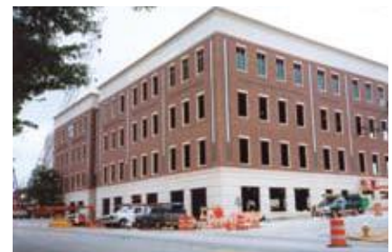
Day 44 — Structurally and architecturally dry.
