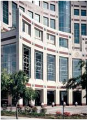
Panels on the Shriners Hospital for Crippled Children, Sacramento, Calif., are 6 in. thick and have a horizontal band of 1 1/4 in. granite attached with one anchor per 2 ft 2 . Architects: Odell Associates; and Associate Architect: HDR.
