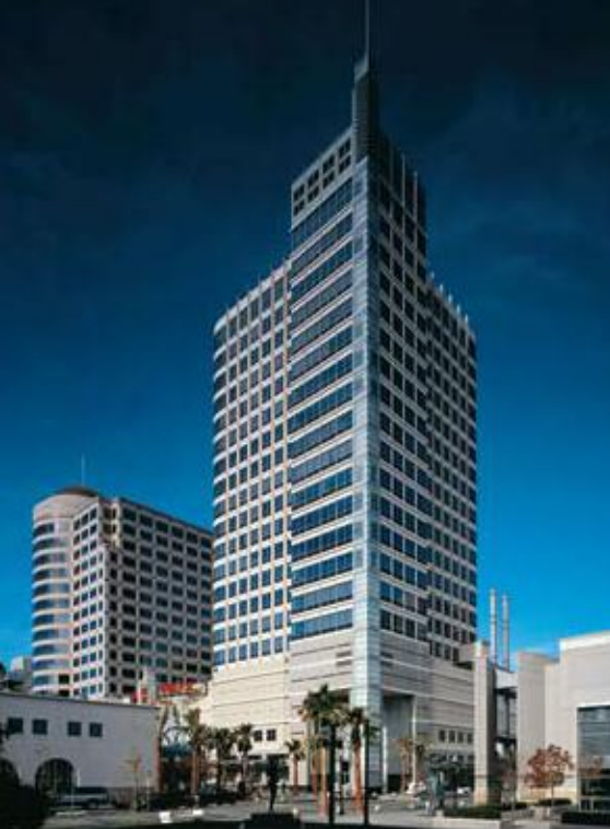
Recalling Art Deco architecture, the Esquire Plaza office tower and mixed-use building in Sacramento, Calif., takes its design cue from the two existing theater façades incorporated in the building. Precast concrete panels on the lower levels and GFRG on the upper portion made the highly articulated façade possible at an affordable cost. Architect: HOK/SF; Photo: Ed Asmus Photography.
