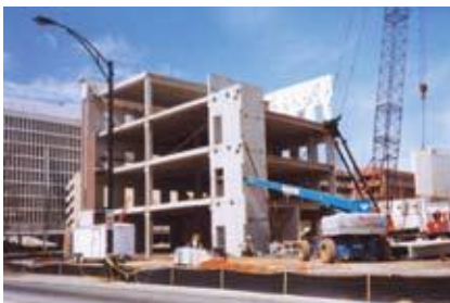
Day 15 — Interior shear walls.
