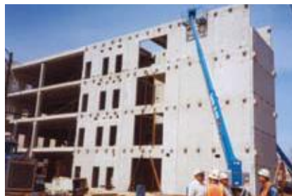
Day 25 — Shear structure.
