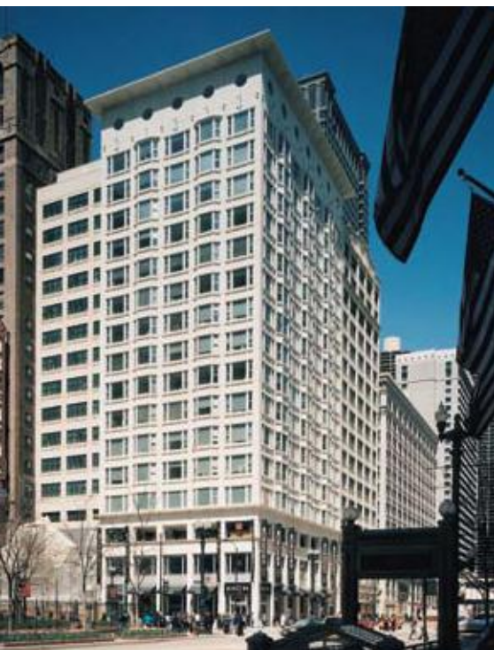
Located in downtown Chicago, Ill., the new residence hall for the School of the Art Institute is clad in GFRG panels, which emulate the look of the Windy City's historic buildings finished in terra cotta. The dormitory is composed of two connected buildings and a rear link. Architect: Booth Hansen Associates Inc., Chicago; Photo: ©Brian Fritz Photography.
