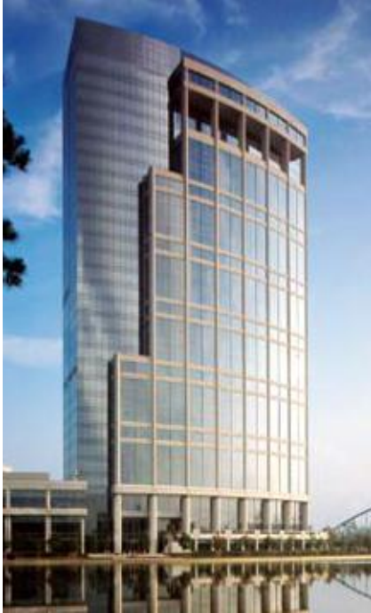
The Anadarko Tower located in The Woodlands, Tex., was clad with light and medium sandblast, textured precast panels composed of a single-face mix design. Some of the panels were supplemented with thermal finished Luna Pearl granite insets. The mix was composed of 100 percent white portland cement, coarse aggregates, fine aggregates, and pigment. Photo: Gensler.
