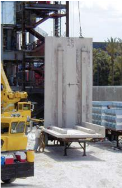
The 6-in.-thick x 22-ft-tall panels were reinforced with ribs spaced 6 ft apart.
