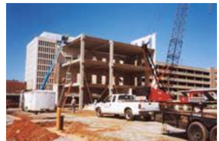
Day 7 — Building begins taking shape.
