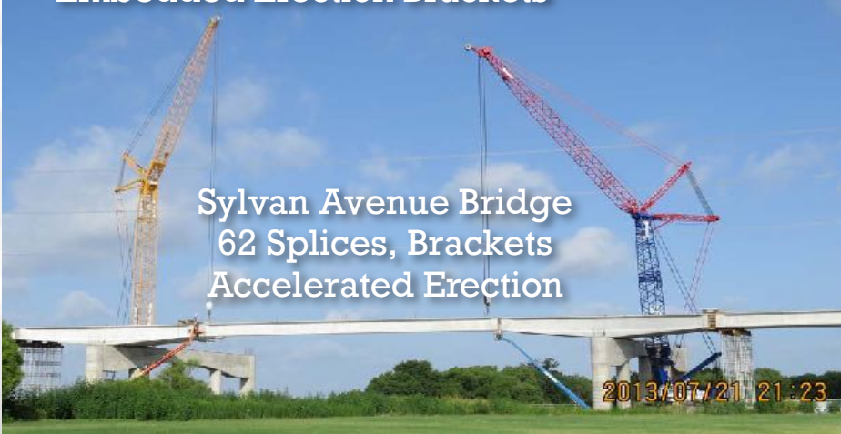
Embedded Erection Brackets
