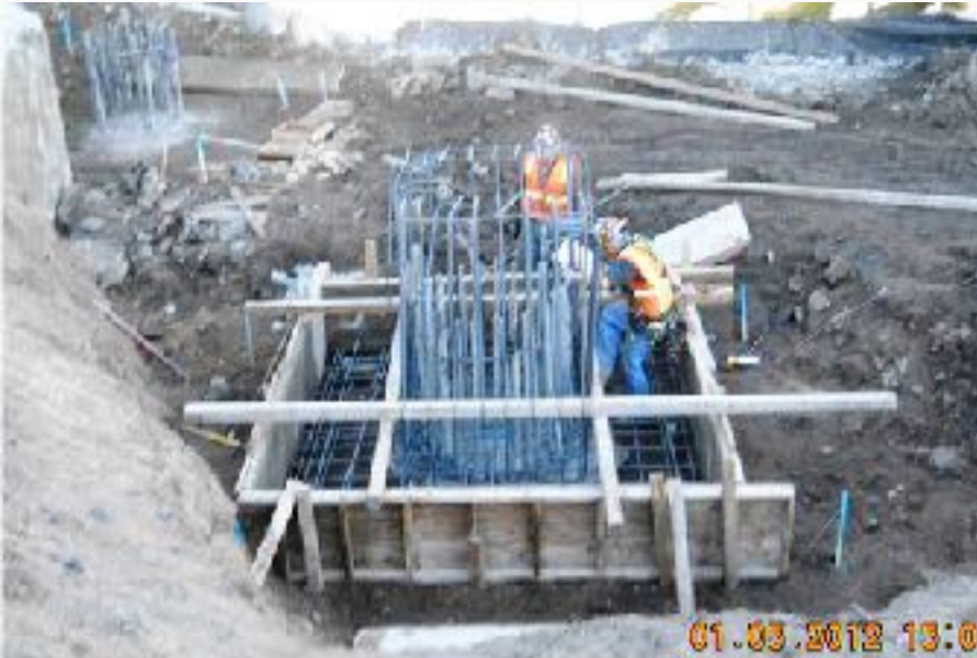
Site Cleared after Demolition. Drilled Shafts Installed
