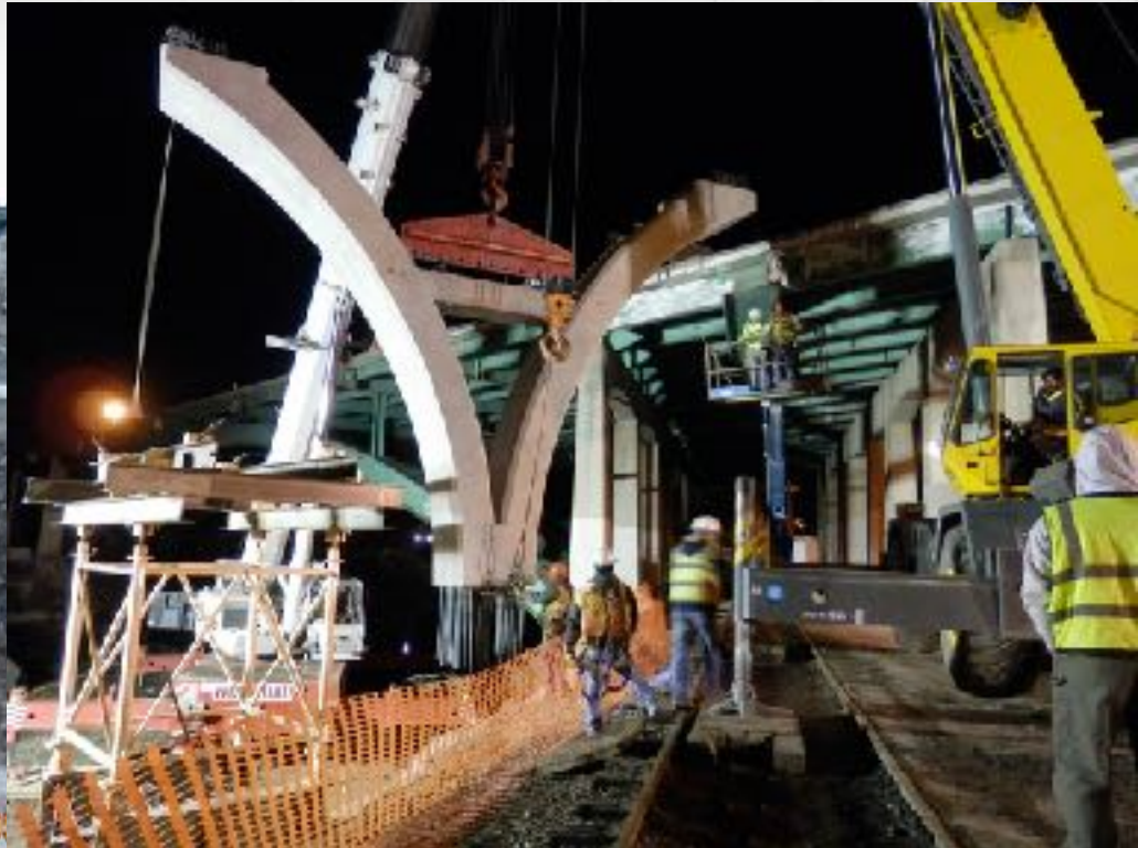
Precast Piers moved to Site Erected in one shift with single crane.
